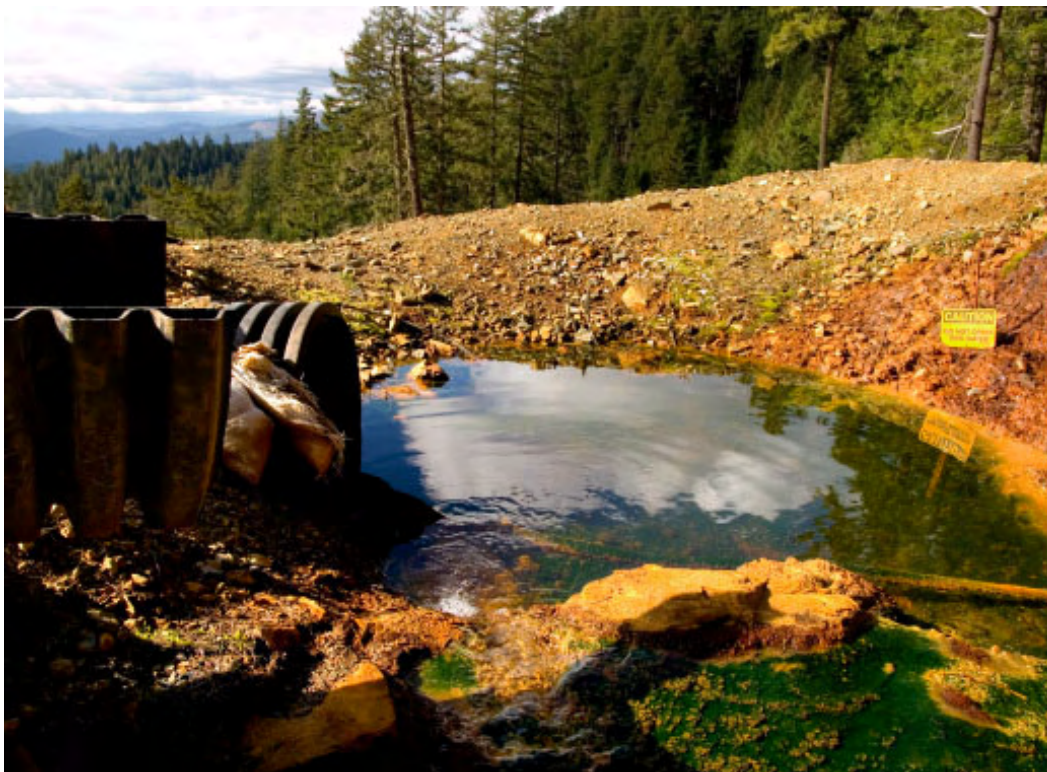
The Formosa Mine in SW Oregon is a toxic Superfund Site and has polluted many miles of waterways. More info at: https://cumulis.epa.gov/supercpad/SiteProfiles/index.cfm?fuseaction=second.Cleanup&id=1002616#bkgground
