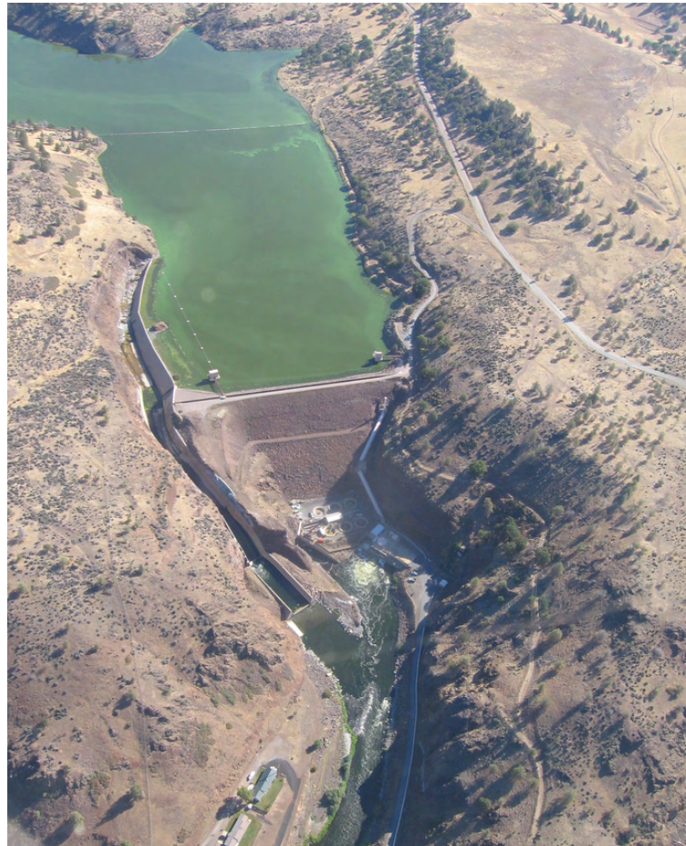
Aerial view of a dam and reservoir on the Klamath River system. Stagnant water behind dams can reach higher temperatures than free-flowing streams, which often leads to toxic algae blooms as seen here.
